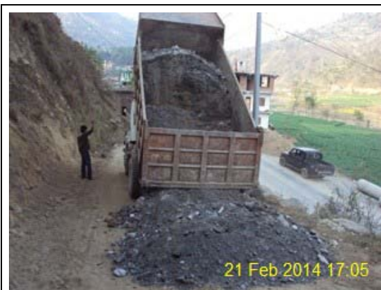
Muck laying on access road to Army Camp bunker at MPB
