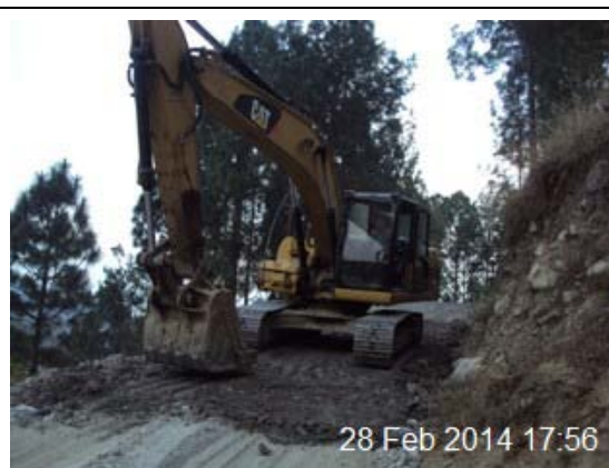
Muck spreading by excavator
