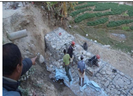
Gabion protection work at Ch. 20+790m
