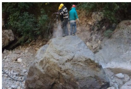
Drilling of big boulders at Headworks
