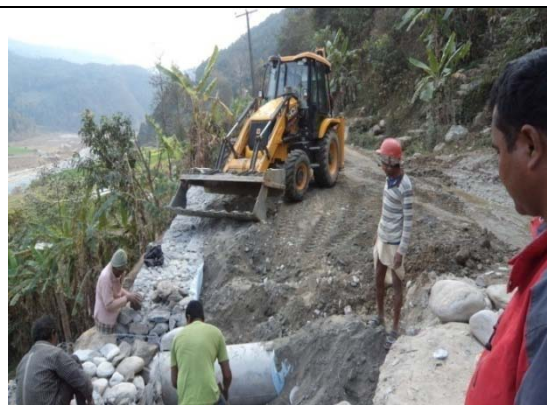
Concrete pipe of 450 mm diameter were installed at Ch. 20+790m & Ch.20+900m
