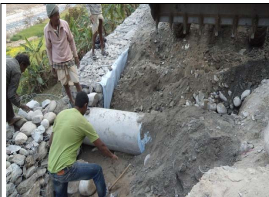
Concrete pipe of 450 mm diameter were installed at Ch. 20+790m & Ch.20+900m
