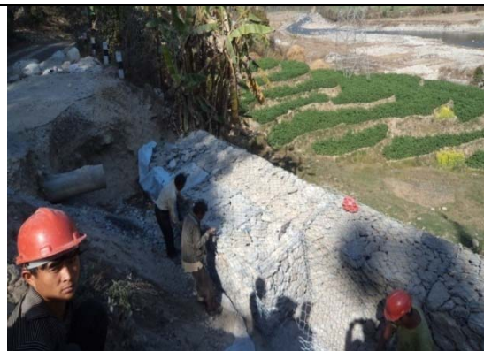
Gabion protection work at Ch. 20+790m
