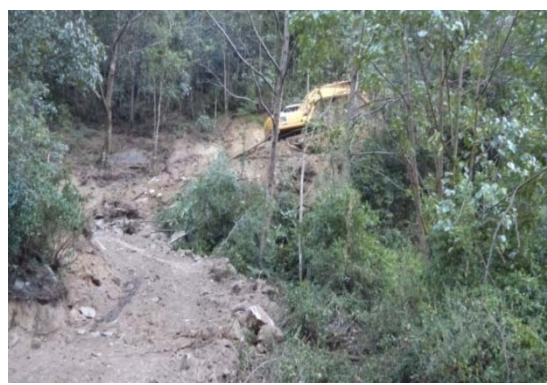
Access Road Track opening for open cut excavation works at Headworks
