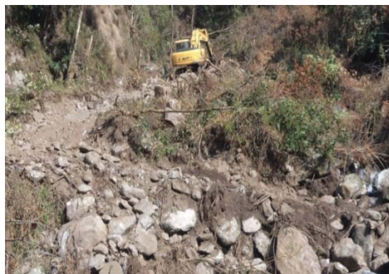
Access Road Track opening for open cut excavation works at Headworks
