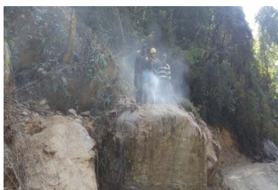
Drilling of big boulders at Headworks
